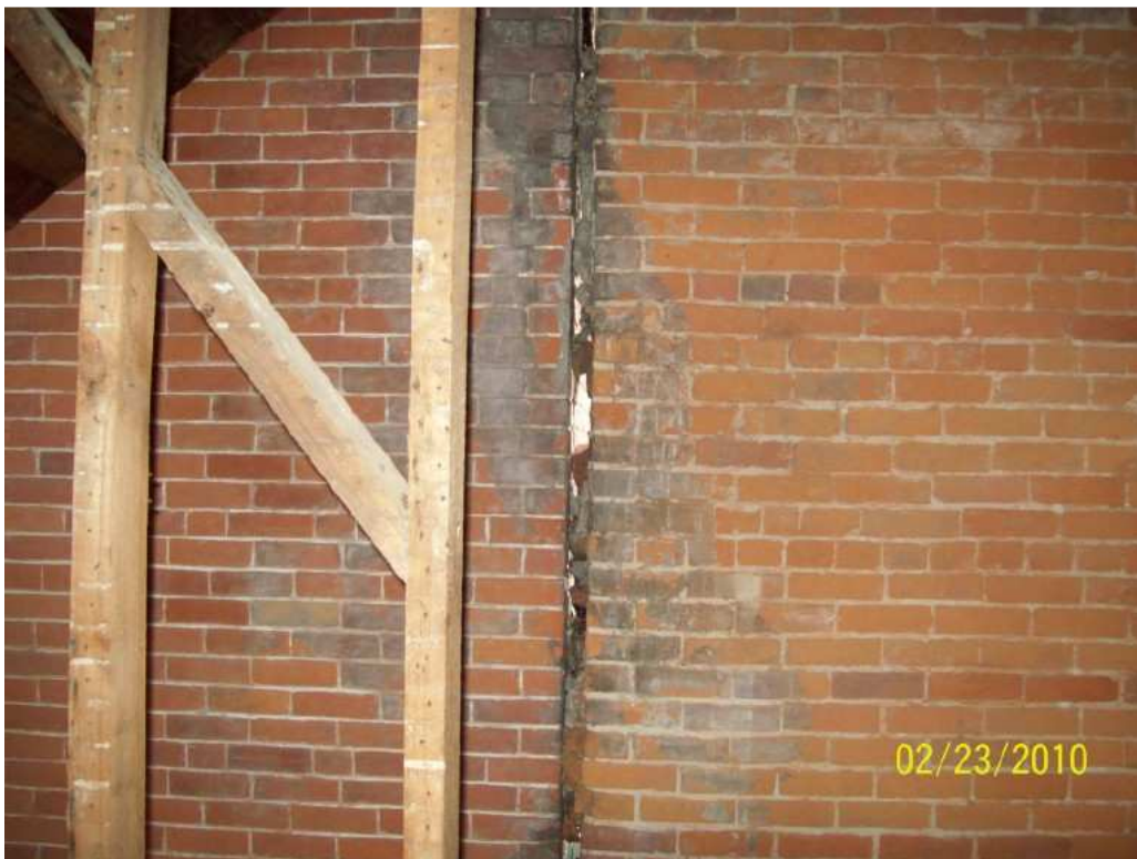
10. Spreading Gap in Wall at 2 nd Floor
