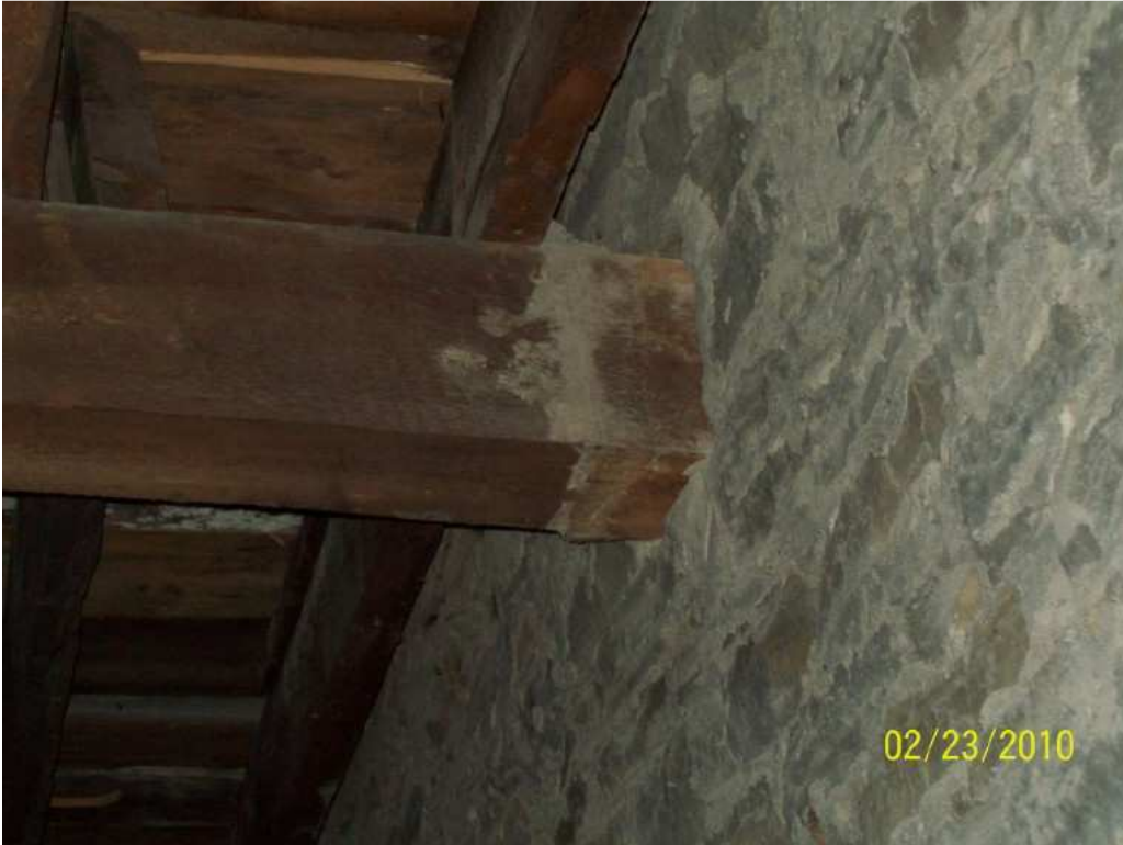
13. Floor Beam Pulled Out From Wall at Basement Floor Structure
