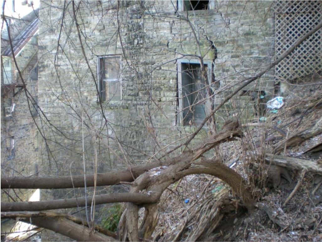
7. Building Wall Cracks at North Wall, Sub-basement Level
