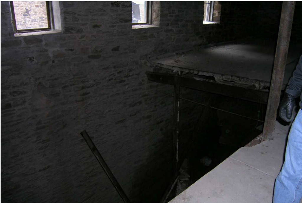
14. Collapsed Sub-Basement Floor
