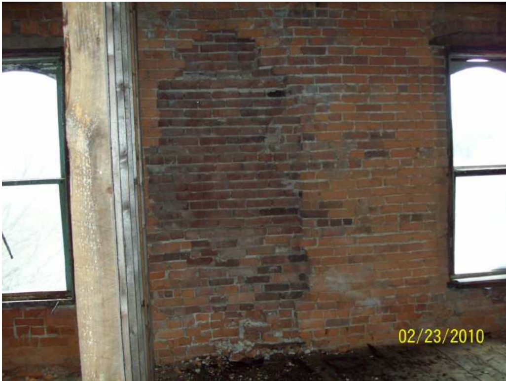
9. Failing back wall at 3 rd floor
